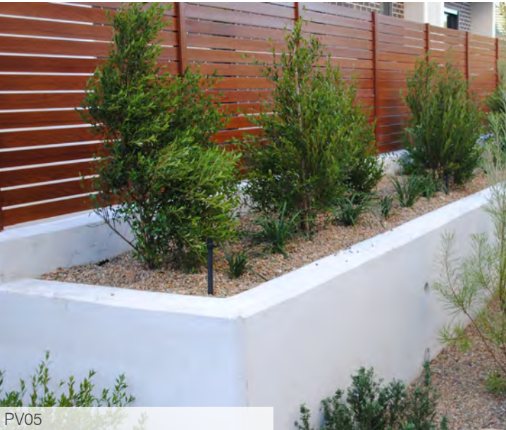
PV05 Insitu Concrete Planter Wall (180mm thick x varied heights
